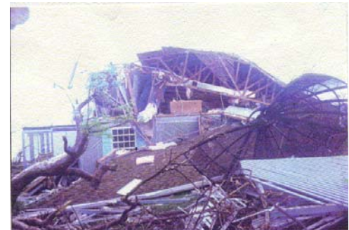
Destruction of expensive timber framed residence (Bahamas)
